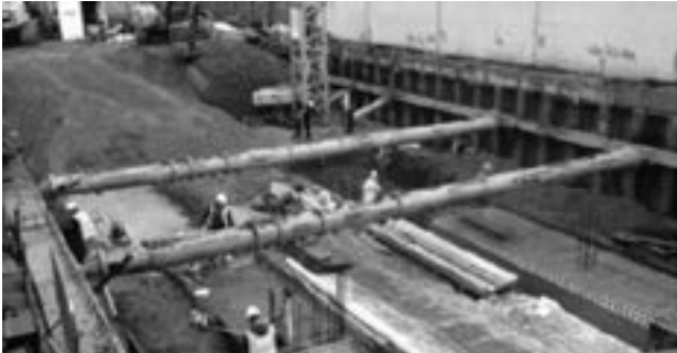
Example of temporary works on a construction site
